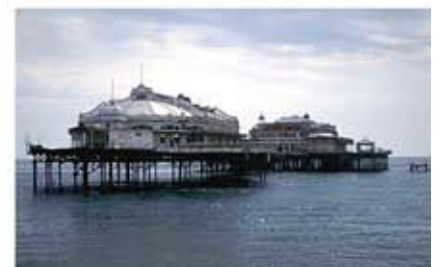
West Pier, Brighton (UK)
